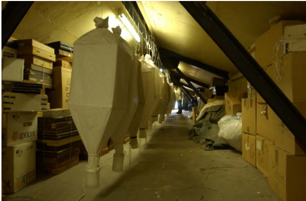
Fig 1. Winkler bags hanging in roof space.
